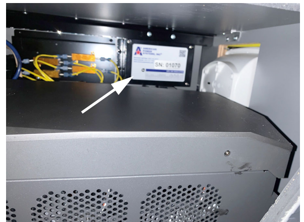
The regulator is located to the back. (The arrow is pointing to the LED indicator located on the APS. Reverse all steps to return panel to the original position. -Typical View
