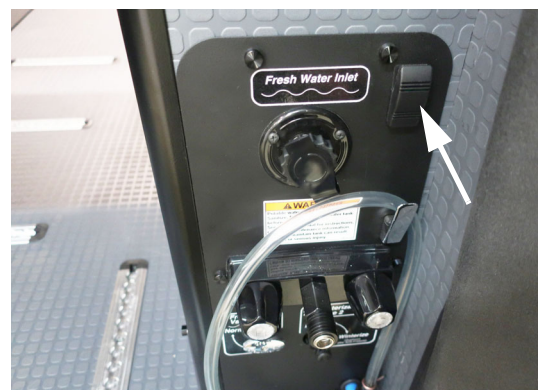
Pump switch -Typical View
